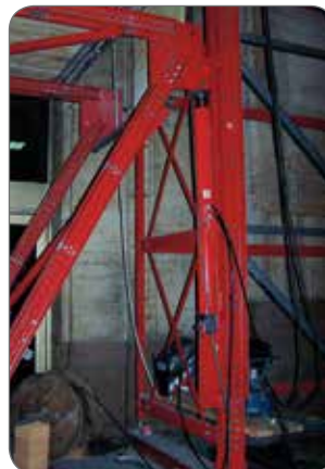
Push cylinders to move decks for building renovation operations.
