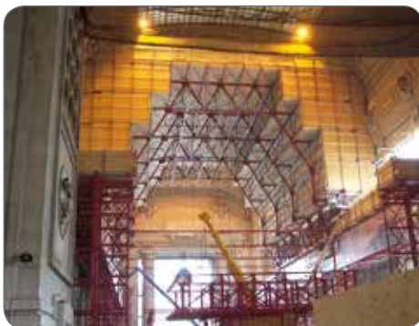
Push cylinders to move decks for building renovation operations.
