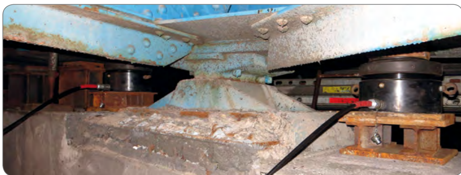
Cylinders to lift structures.
